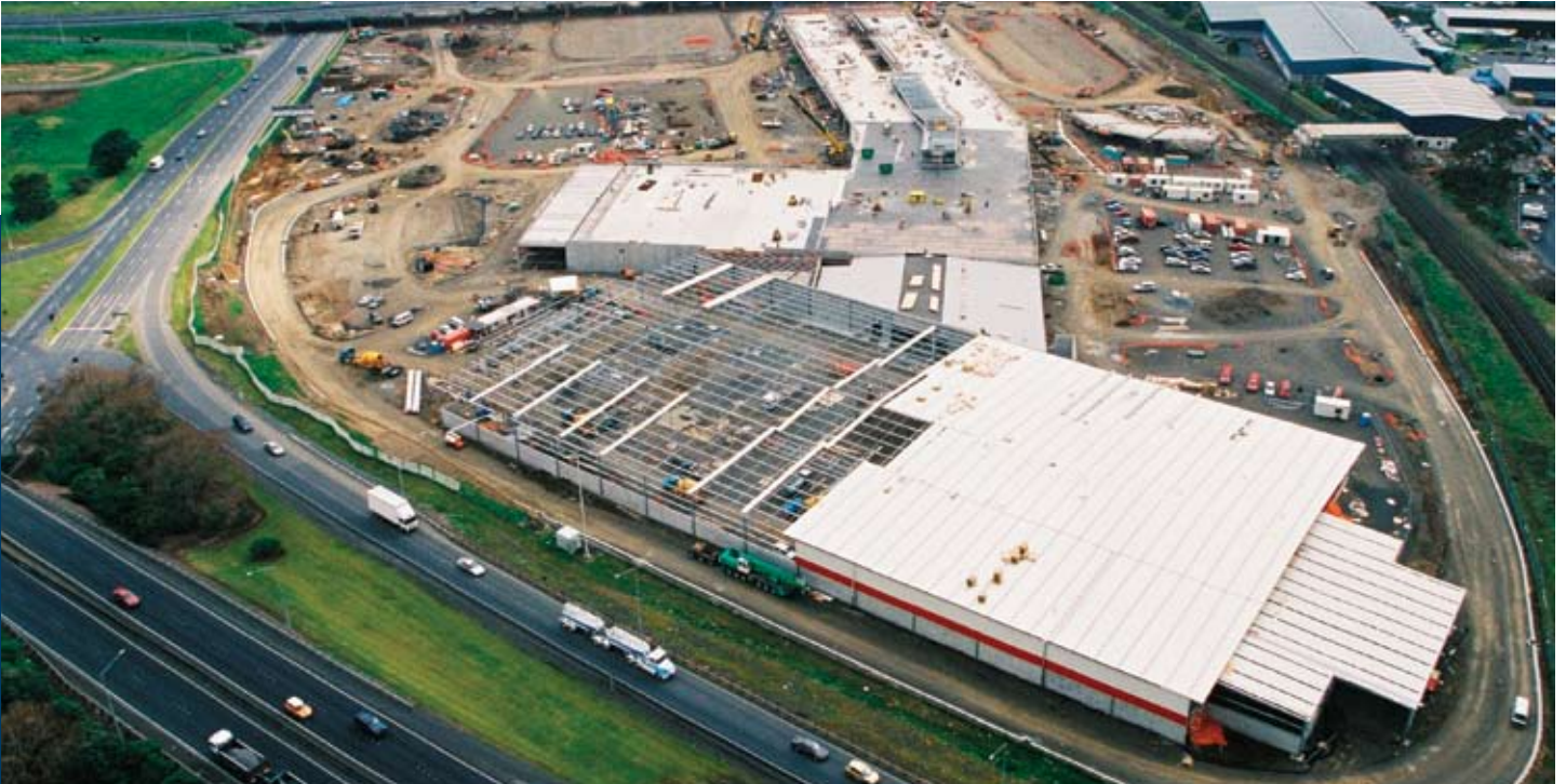
ABOVE: The Warehouse, Foodtown and main mall construction.
