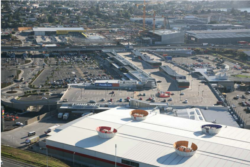
View North – Stage I & II
