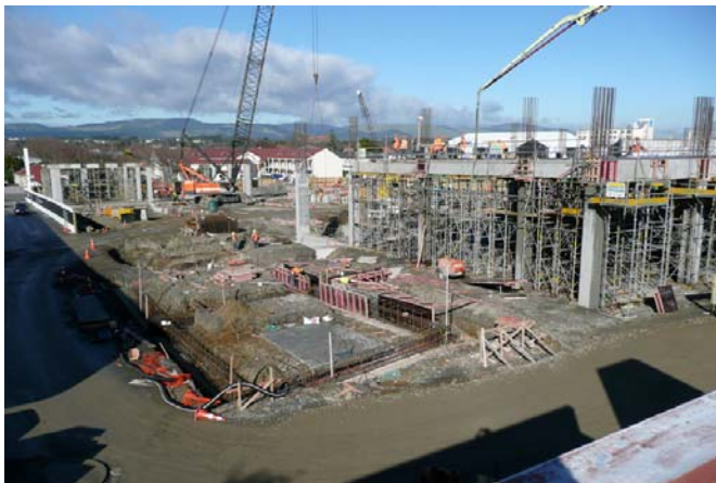
Construction progress on multi-storey carpark The Plaza Shopping Centre, Palmerston North
